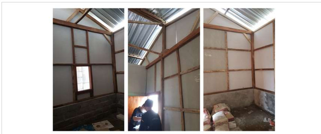
Figure 11. The construction of Huntara's wooden frame
