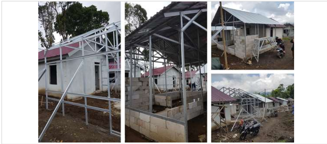
Figure 10. The construction of Huntara
