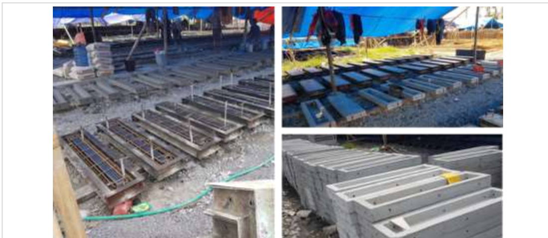
Figure 9. In situ precast for Huntap structural elements
