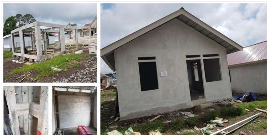
Figure 12. The construction of permanent housing (Huntap)
