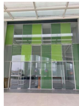
Gambar 6. Tampak Depan Existing Ruang KKI [Sumber: Penulis, 2022]
