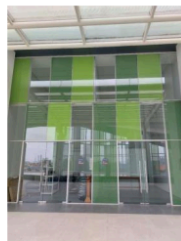
Gambar 6. Tampak Depan Existing Ruang KKI [Sumber: Penulis, 2022]
