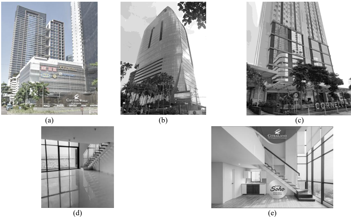
Fig.3. Some loft office buildings in Surabaya (a) Ciputra World Surabaya Vie Loft SOHO (b) Satoria Tower (c) exterior Cornell Apartment and SOHO (adapted from https://www.google.com/maps/place/ ) (d) interior of Ciputra World Surabaya Vie Loft SOHO (e) interior of Cornell Apartment and SOHO ( https://citralandsurabaya.com/soho-cornell-corner/ )
